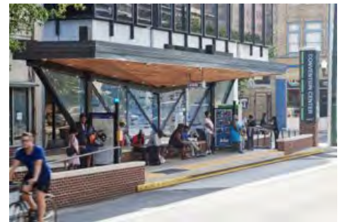
Enhanced station example. GRTC (VA) Pulse station (Source: Kimley-Horn)
